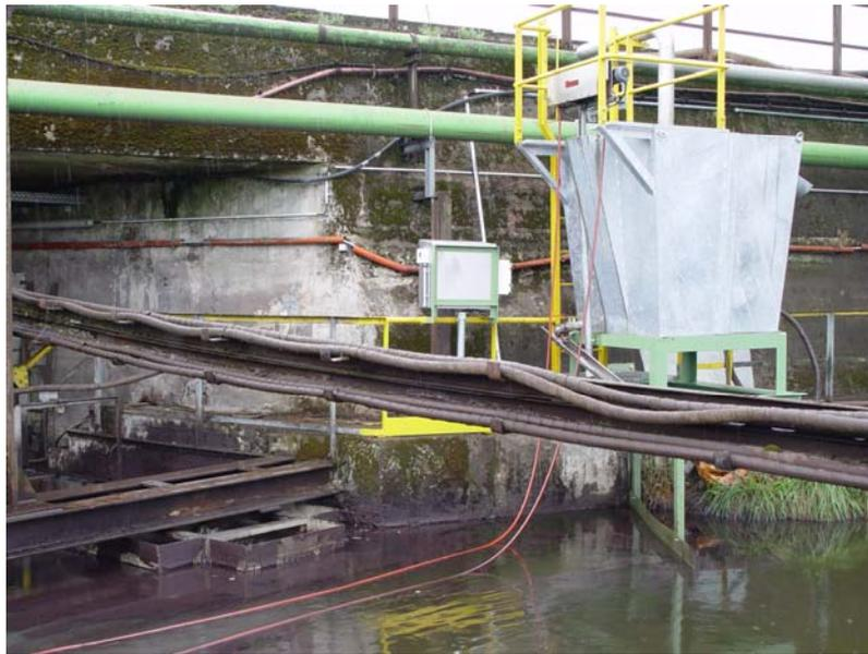
**oil skimmer S 100 at cooling water basin with more than 1000 m<sup>2</sup> surface**
