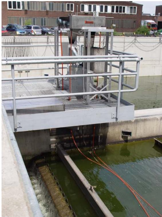
oil skimmer model S 100 mounted at longitudinal clarifier
