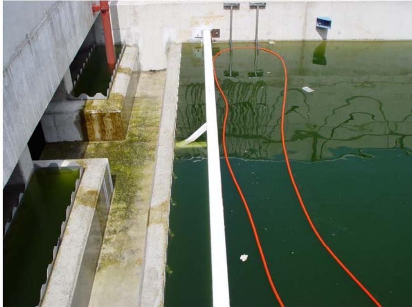
oil collector tube floating on longitudinal clarifier
